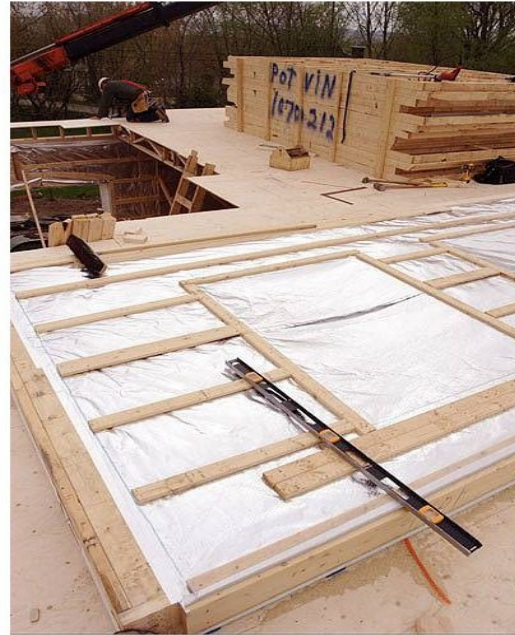
Prefabricated walls built in a factory, shipped by truck and lifted into place by a crane
