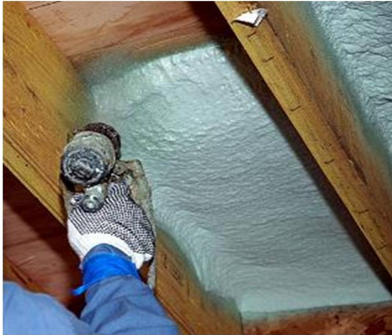
Spray foam insulation is available in two types: Closed cell at R-6.5 per inch and open cell
