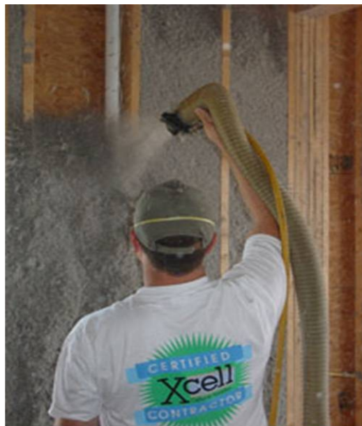
spray cellulose insulation
